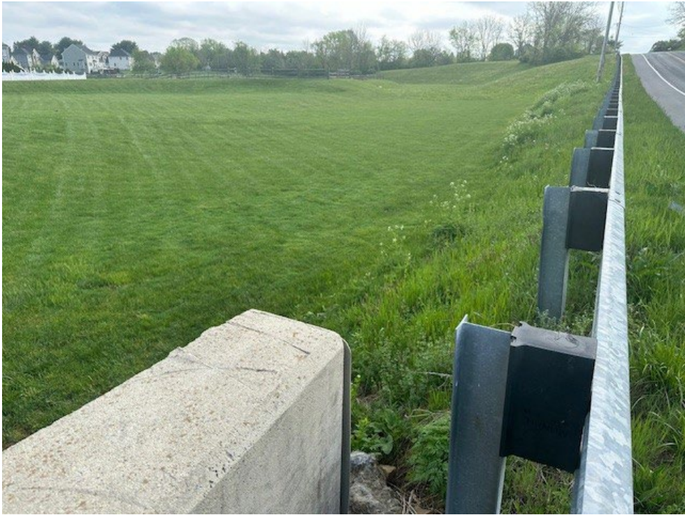
Looking North at Swale Headwall
