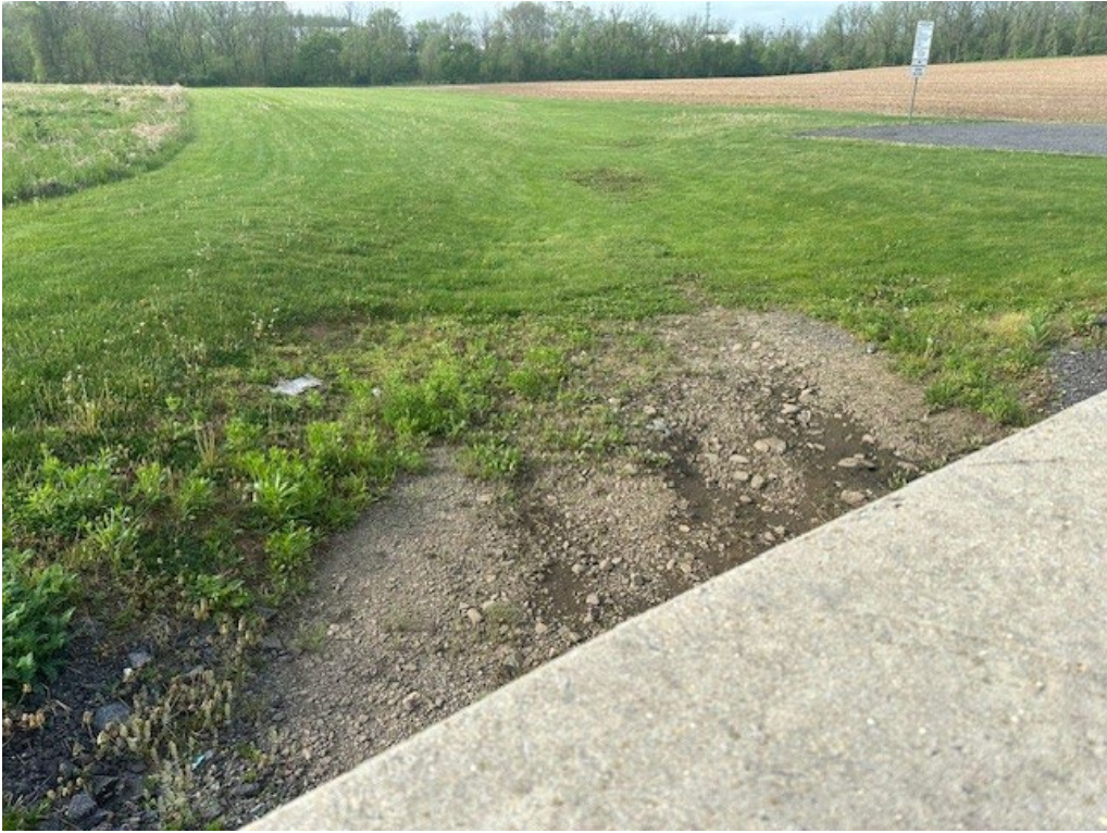
Looking South at Swale Headwall
