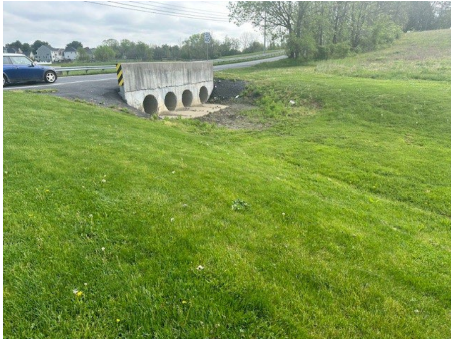
Swale at South Side of Headwall
